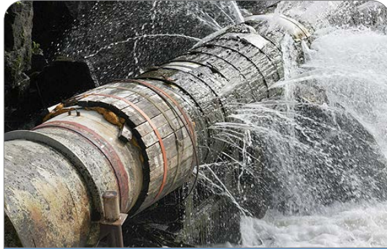
Significant 'lost water' and supply inefficiencies
