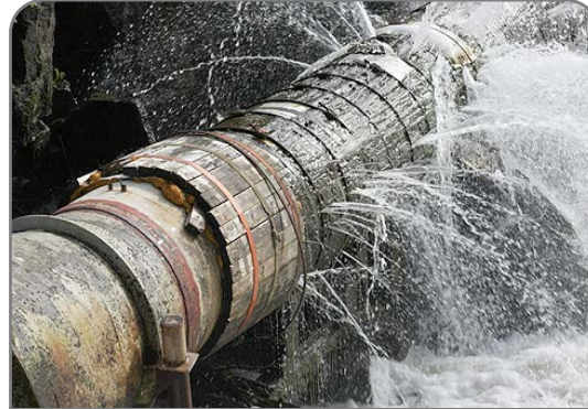
Significant 'lost water' and supply inefficiencies
